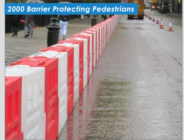
2000 Barriers On Site
