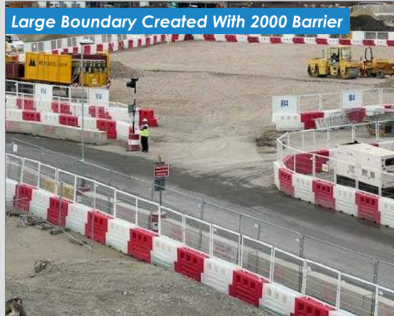
Protecting Temporary Works
