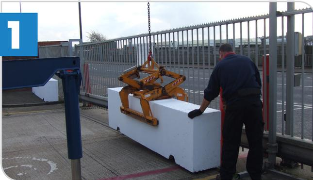
Plan where you want the barriers to be positioned and position close to their final position using a forklift truck.
