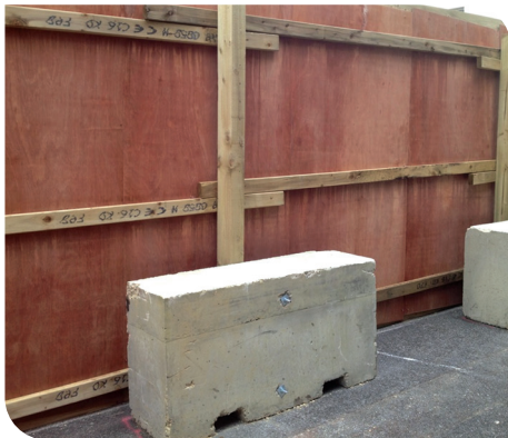
3m concrete barriers in situ as timber hoarding ballast
