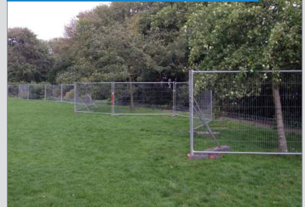
Anti-Climb Fencing Protecting Tree Line
