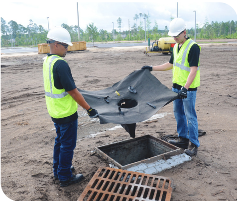
Site workers preparing Drain Guard
