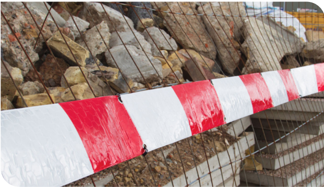
FenceBrite Strips attached to temporary fencing
