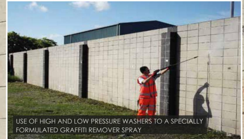
USE OF HIGH AND LOW PRESSURE WASHERS TO A SPECIALLY FORMULATED GRAFFITI REMOVER SPRAY
