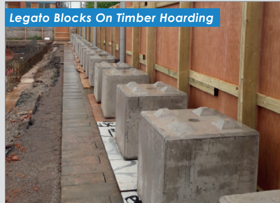
1.5m Concrete Block Used For Ballast
