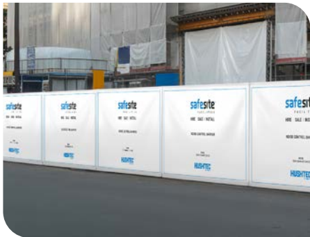
Hushtec 3.5m Performance Acoustic Barriers installed on scaffolding site
