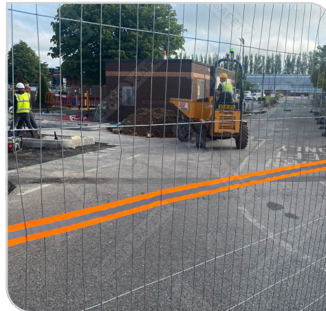
Fence Webb tape attached to fencing
