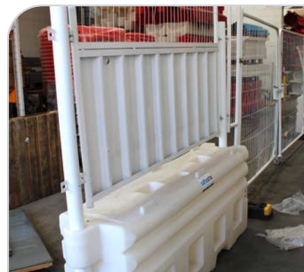
Half hoarding & fence next to vehicle gate
