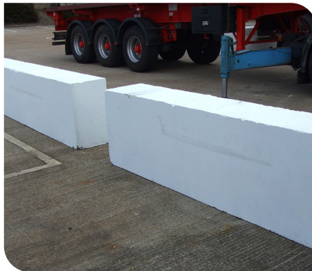
Offloading of 4m concrete barrier
