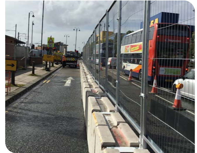
TVCB's creating safe zone for workers
