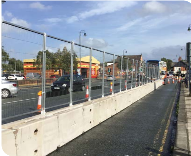
TVCB's with fence securing highway
