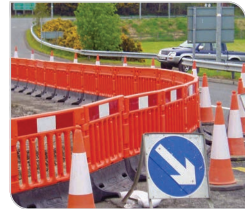
StrongWall used roadside
