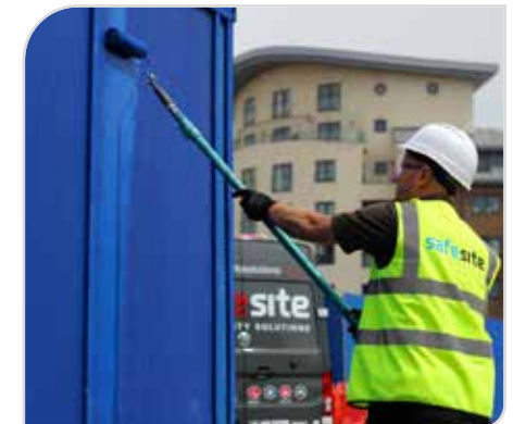
Face side of hoarding can be painted
