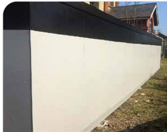
Hoarding with anti-climb paint
