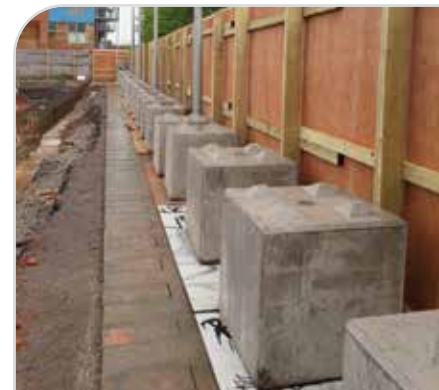
Legato blocks on timber hoarding
