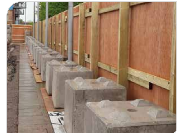
Legato blocks supporting hoarding
