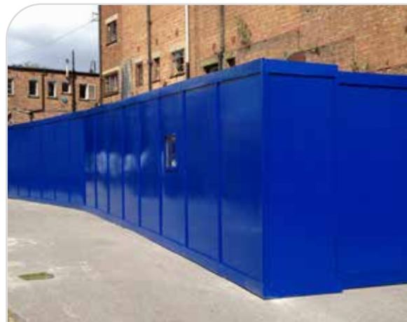
Hoarding painted in company colours
