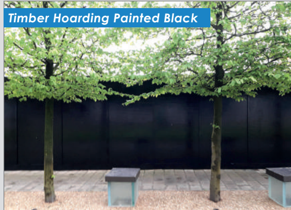
Timber Hoarding In Chichester
