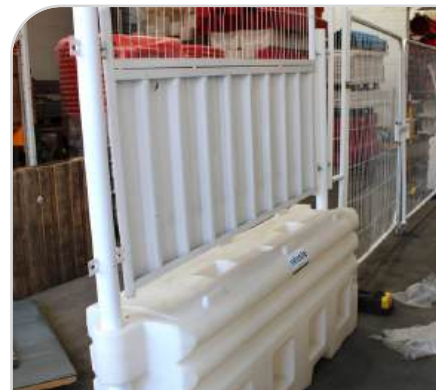
Half hoarding & fence next to vehicle gate
