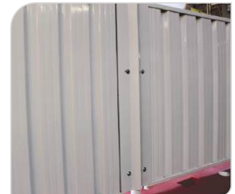
Hoarding infill panel
