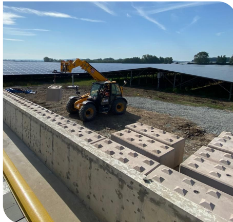
Legato Blocks on site
