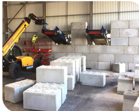
Legato Wall Being Constructed
