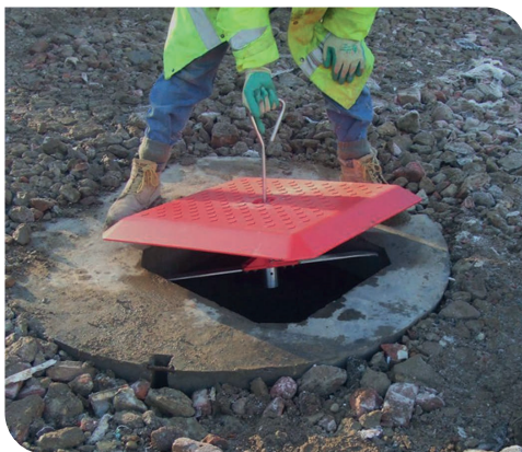
Cover being installed & locked
