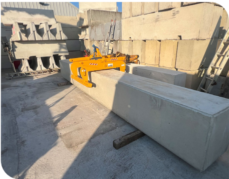
6m concrete barrier being lifted with crane
