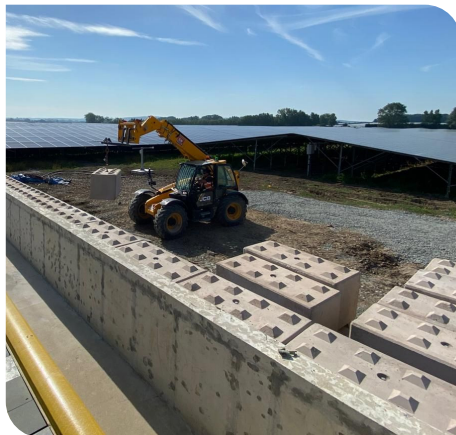
Legato Blocks on site
