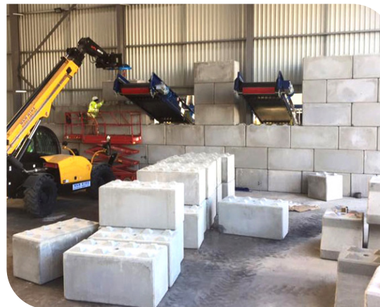
Legato Wall Being Constructed
