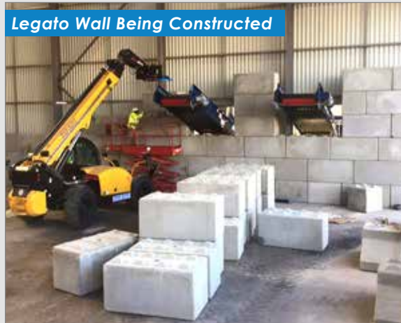
Legato Blocks Form Dividing Wall
