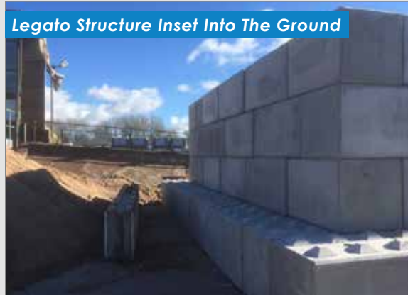
Storage Bay Constructed From LG8 Blocks
