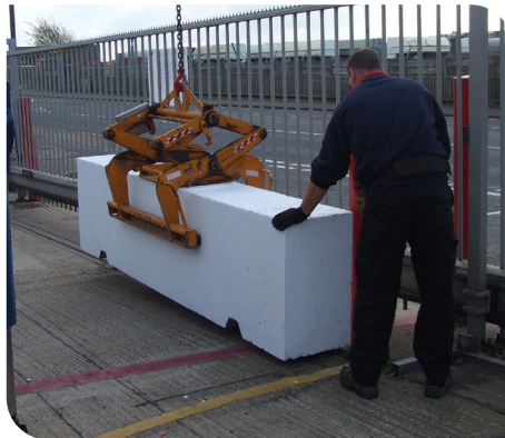
Offloading of 3m concrete barrier
