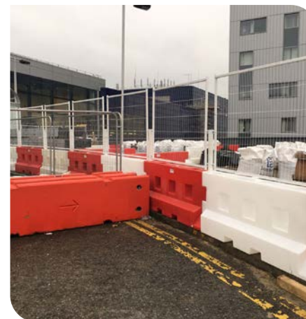
GB2 securing building materials
