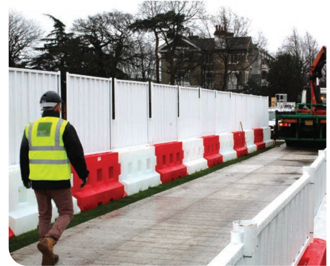
Full & half hoarding securing site entrance
