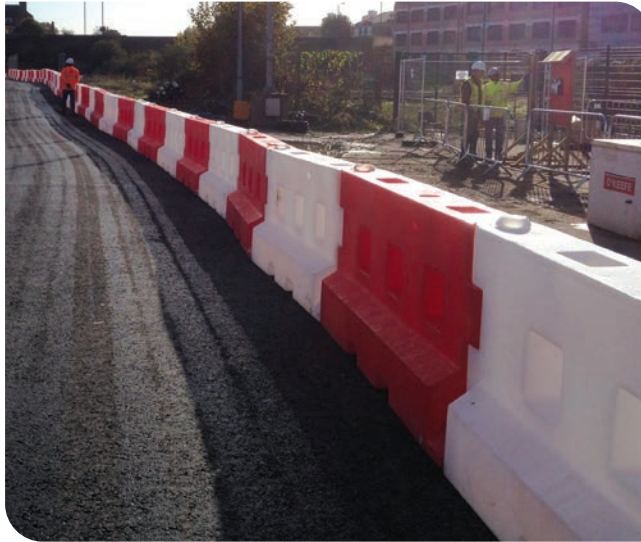
GB2's forming road perimeter on site
