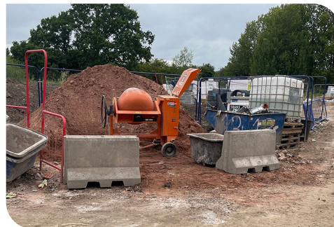
1.2m Concrete Jersey Barriers on site
