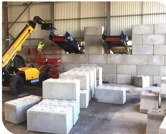
Legato Wall Being Constructed
