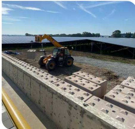
Legato Blocks on site
