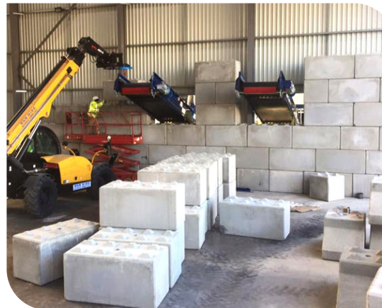
Legato Wall Being Constructed
