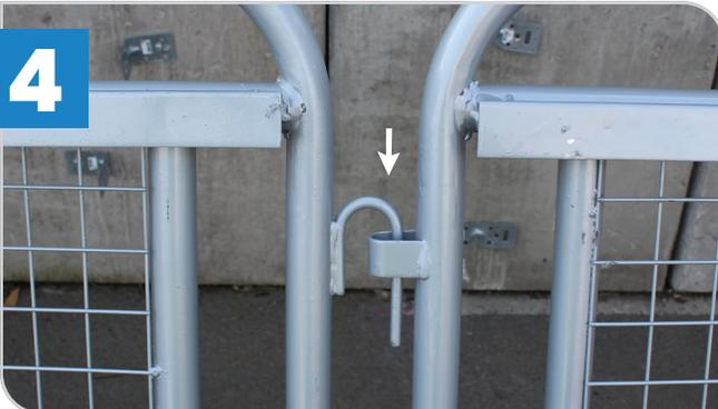
As you position the fence panel in the foot, line up the hook on side of the panel with the loop on the fixed panel.
