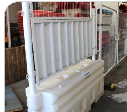
Half hoarding & fence next to vehicle gate
