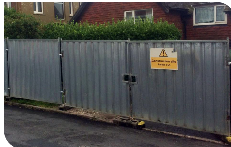
Steel Hoarding Installed with Vehicle Gate
