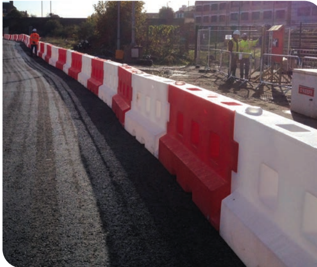
GB2's forming road perimeter on site
