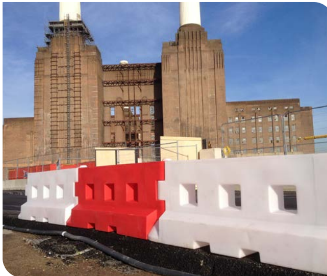
GB2's securing large demolition site
