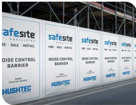
Hushtec 1.2m Performance Acoustic Barriers installed on scaffolding site
