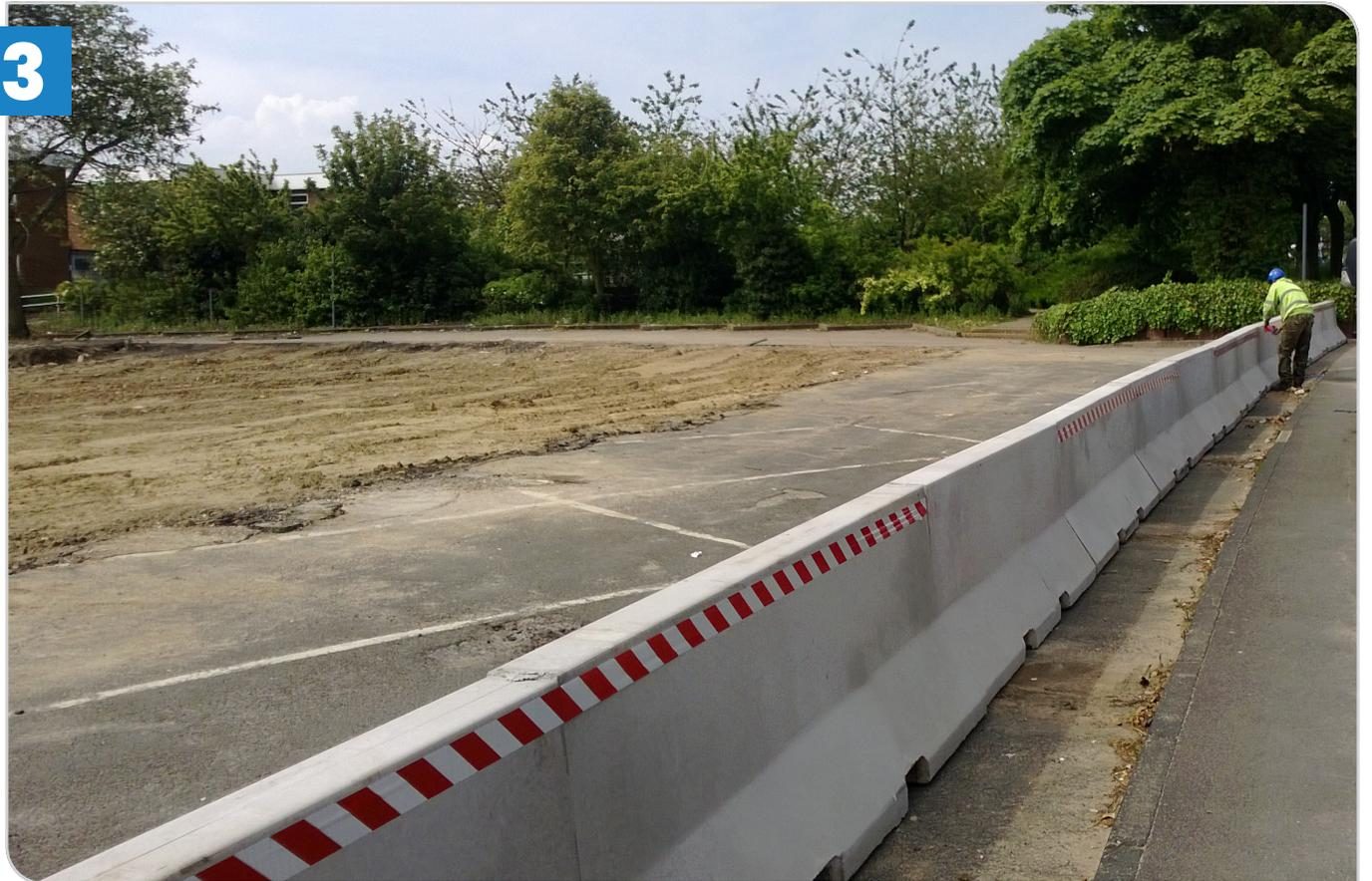
**3** Fix your first barrier in position and butt the second barrier up to the first. The Jersey barriers are designed to interlock and fit together to form a tight join.
