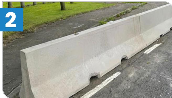
**2** Use forklift truck to position the barriers in the correct place. The distance between the forklift holes on each barrier is 600mm. Each forklift slot 180mm.
