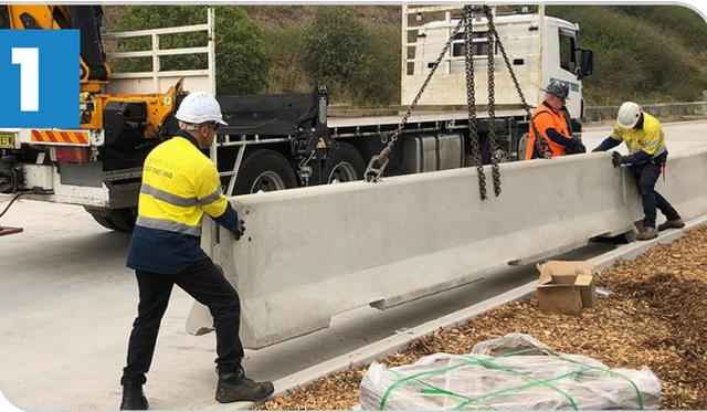
**1** Plan where you want the barriers to be positioned and position close to their final position using a specialist equipment (such as a telehandler).
