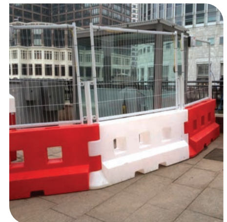
Forming curved perimeter
