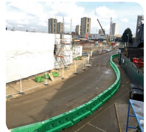
Bending around site perimeter
