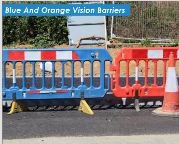
Protection For Fresh Tarmac Being Laid
