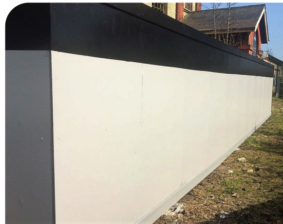
Hoarding with anti-climb paint
