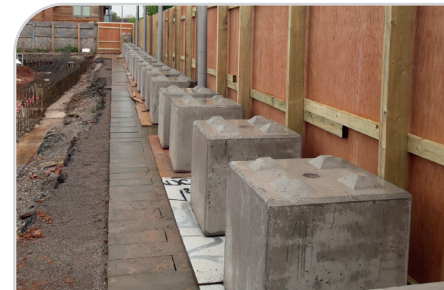
Legato blocks on timber hoarding
