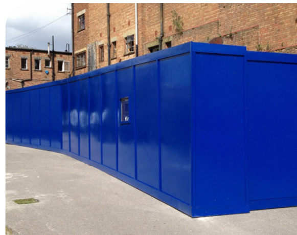
Hoarding painted in company colours
