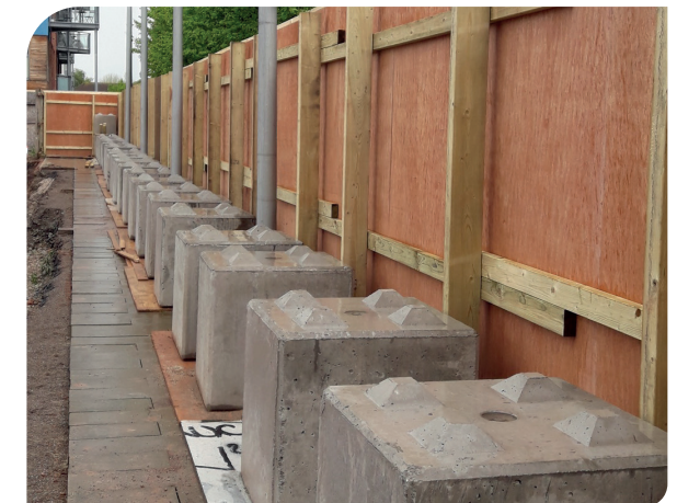
Legato blocks supporting hoarding
