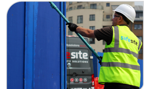
Face side of hoarding can be painted
