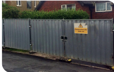
Steel Hoarding Installed with Vehicle Gate
